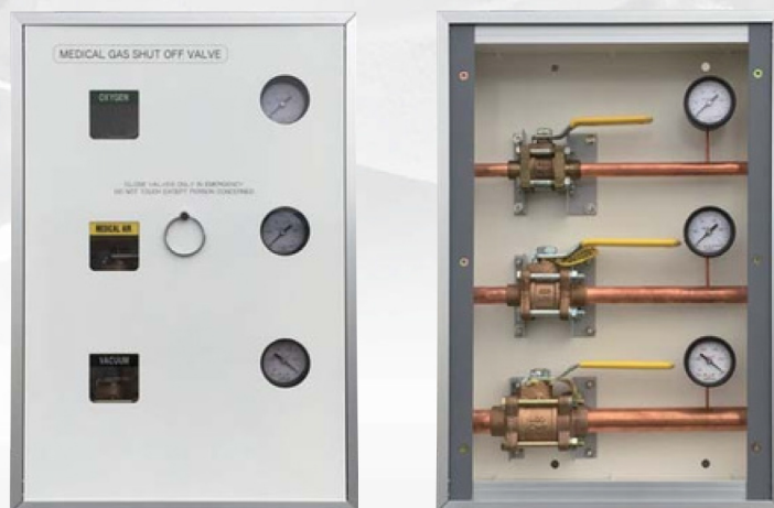
Maximum 7 valves in one box Size of Valve is 1/2"~3"
